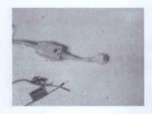
Install the ground wire, then connect the plug to the electrical
