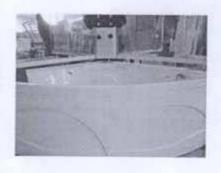
Connect the tub and the glass backboard with screws
