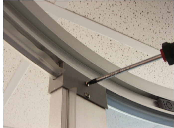
Picture shows top fixing repeat both sides and at the bottom as well
