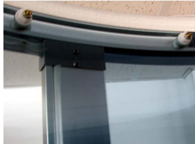
Top door wheels in place note cam adjustment
