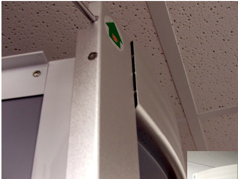
Offering up the top rail to slot into clips
