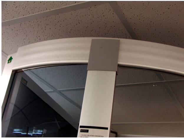
Offering up the top rail to slot into clips
