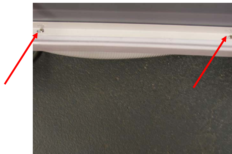
2 x screws placed through bottom of glass frame into shower tray Taking
