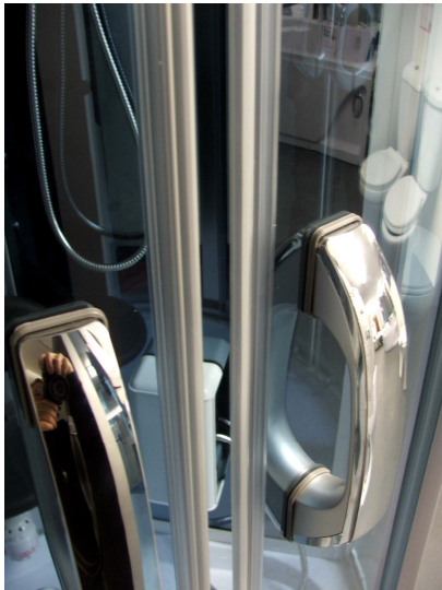
Magnets fitted to doors to attract each other
