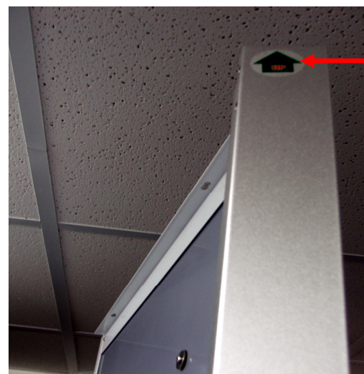
Column showing "UP"
