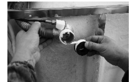
6. Use thread sealing tape to wrap around the drain hole
