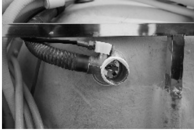
7. Make the thread sealing tape smooth
