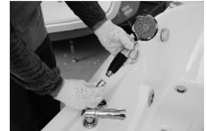
2. Connect the hand shower with the hose into the bathtub in right position as pic. Shows
