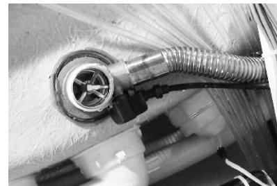
7. Make the thread sealing tape smooth
