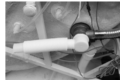
8. Fasten the drain tube
